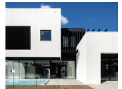
Exterior wall cladding
